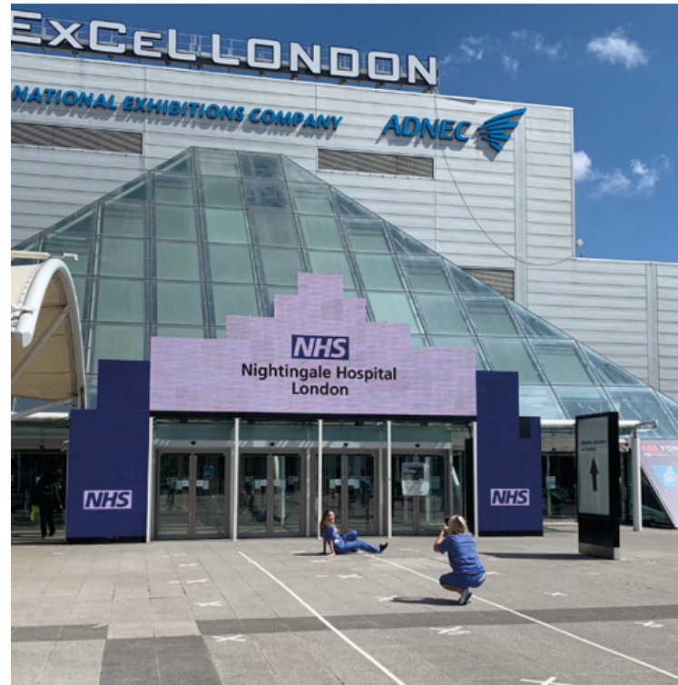
The specially constructed Nightingale Hospital London
